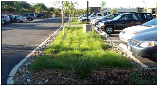
Exhibit Conservation-2. Pervious, Vegetated Areas within Parking Lot (Left) and Street (Right) to Filter and Infiltrate Stormwater
