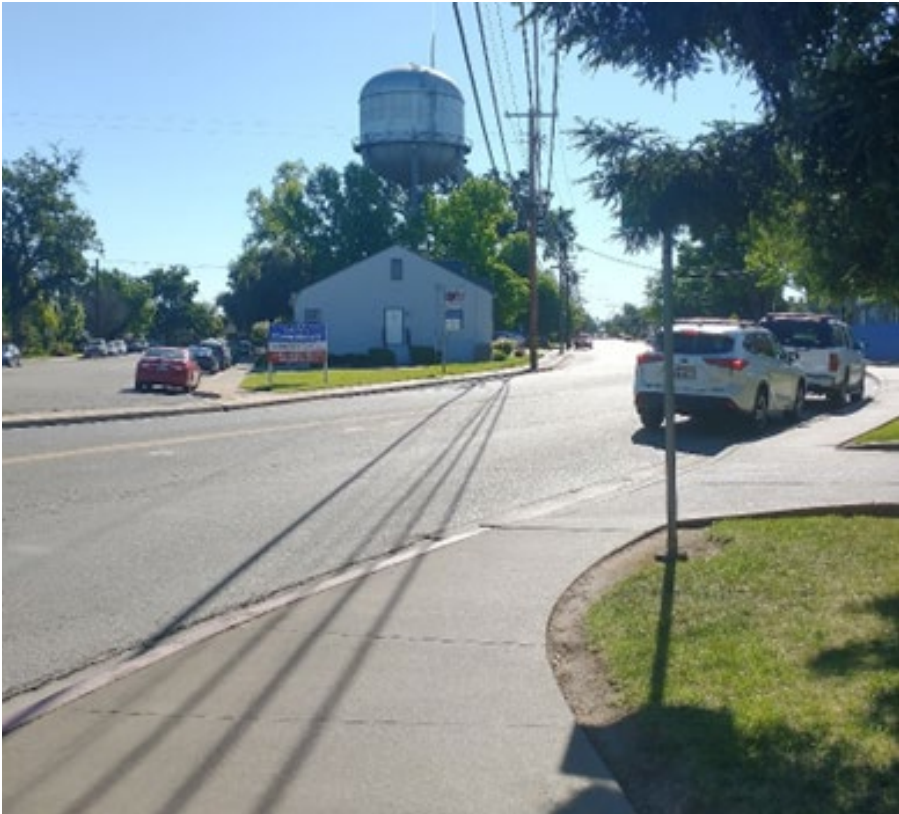
Roadway curvature on Magnolia Street
