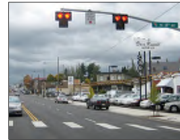
Install Pedestrian Signal
