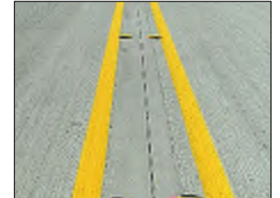
Install raised pavement markers and striping
