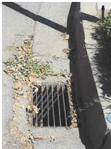
Old drainage grates that were replaced due to hazards to cyclists.
